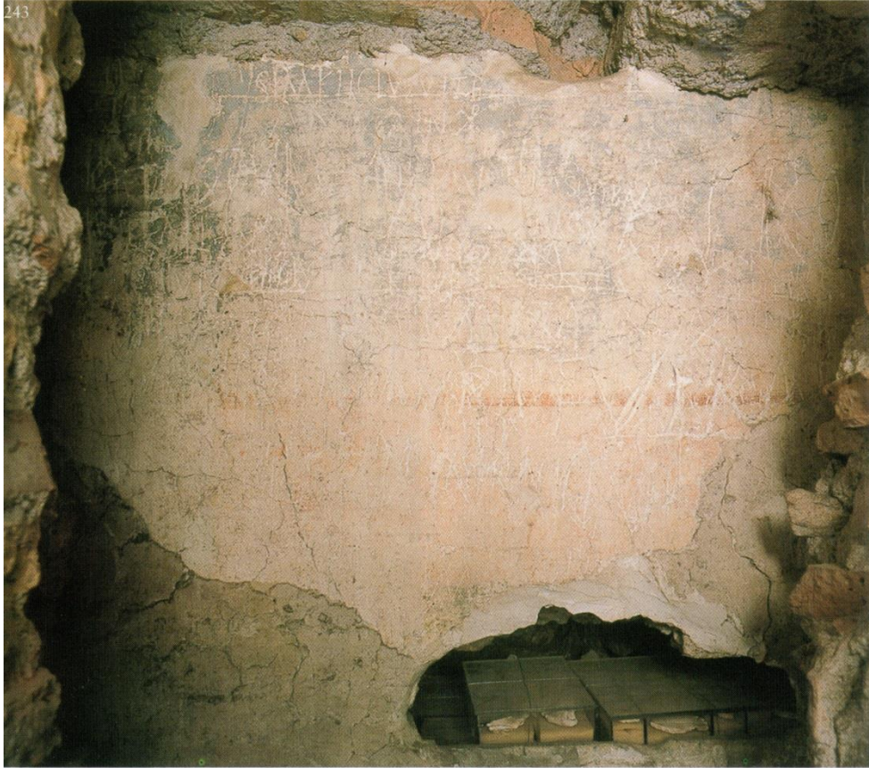
243. Constantinian Memorial - north zone, detail of "Wall G" or "of the graffiti" with a loculus (cavity) made in its interior at the beginning of the 4 th c.
